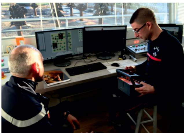
Operators with radio control pendant
